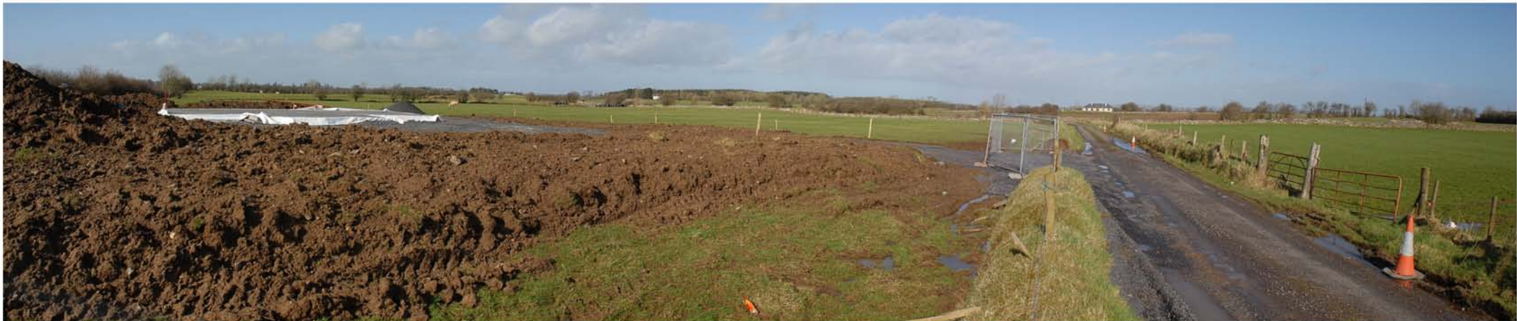
Plate 8: Location of a house under construction near Frenchpark Demesne
