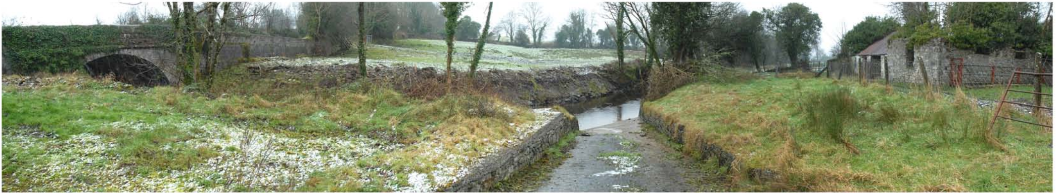
Plate 16: River access point at Cloonfinlough
