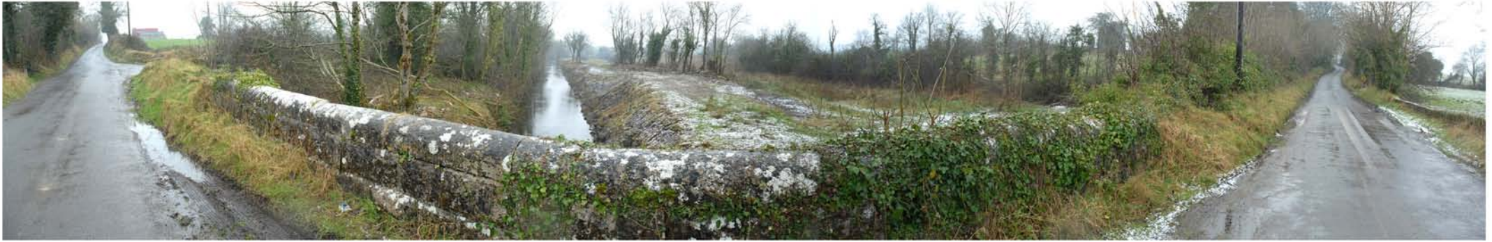
Plate 15: Scramoge River tributary crossing at Cloonfinlough
