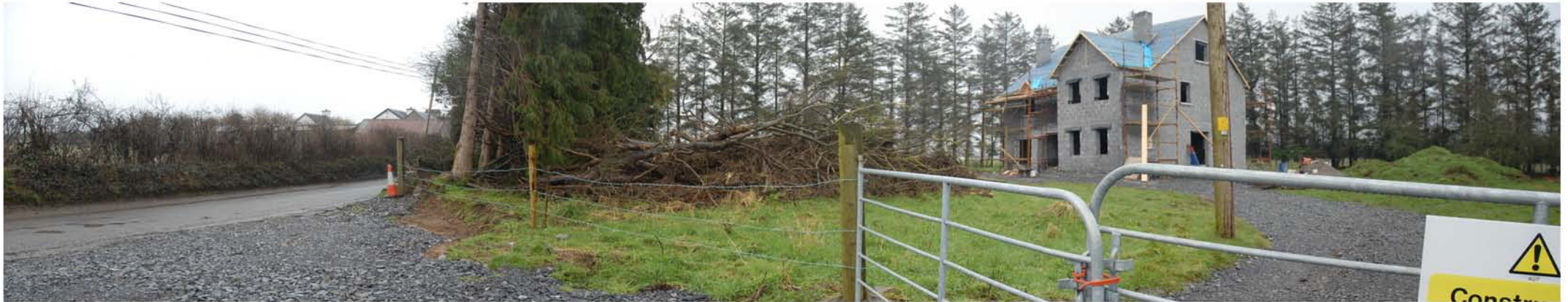
Plate 13: House under construction at Lissaphobble close to Corridors 2A and 2B
