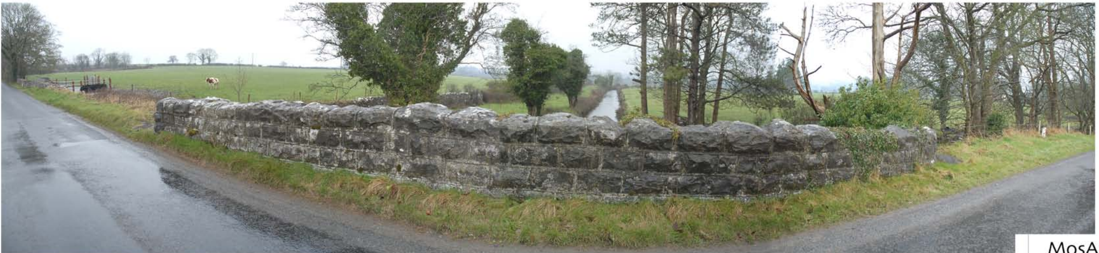
Plate 14: Crossing of Scramoge River tributary near Ballyhammon
